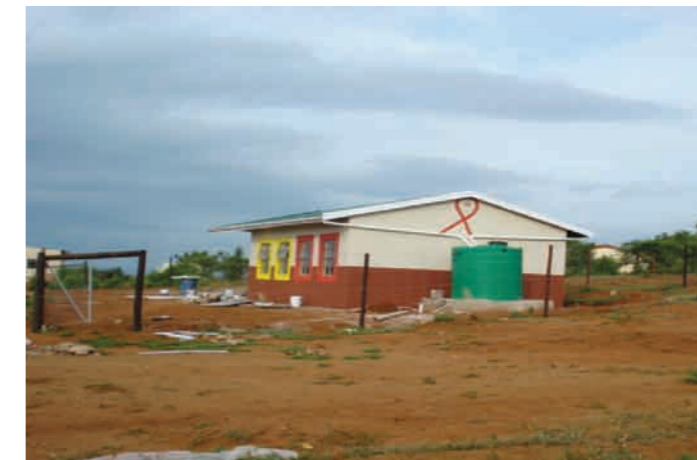
Mbhekeni Crèche with fencing and VIP Toilets
