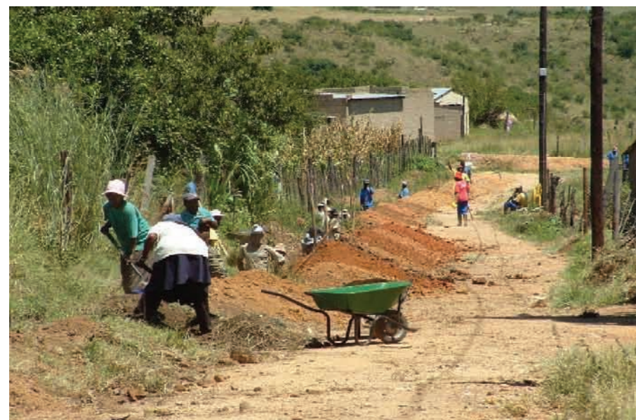
Excavation of a Reticulation Line at Simdlangetsha West Using Local Labour
